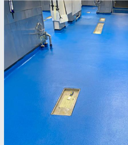
SynDeck flexible, waterproof, anti-slip full resin system, pending scupper grate installation.
