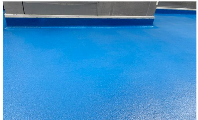
Installed anti-slip galley floor with crack resistant SynDeck flexible, waterproof, full resin system.
