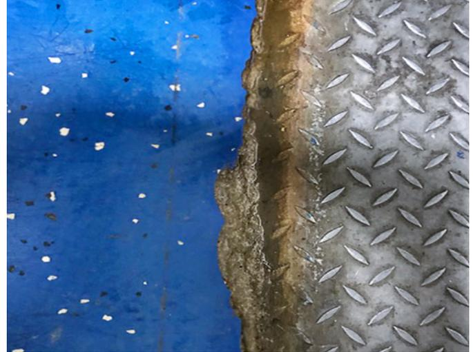
Failed concrete underlayment and coatings with cracks and delamination.
