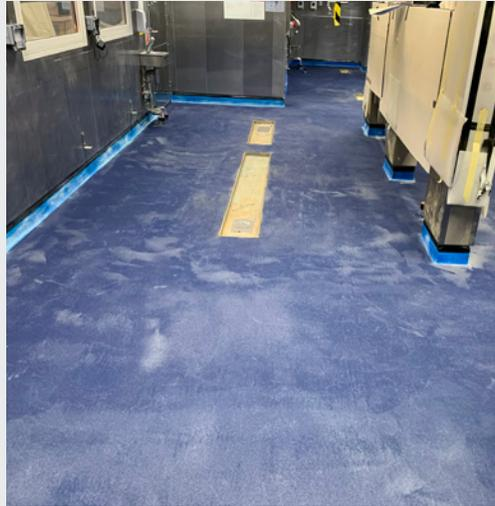
Installed SynDeck Flex IMO flexible, water barrier epoxy with anti-slip quartz broadcast over waterproof resin underlayment.
