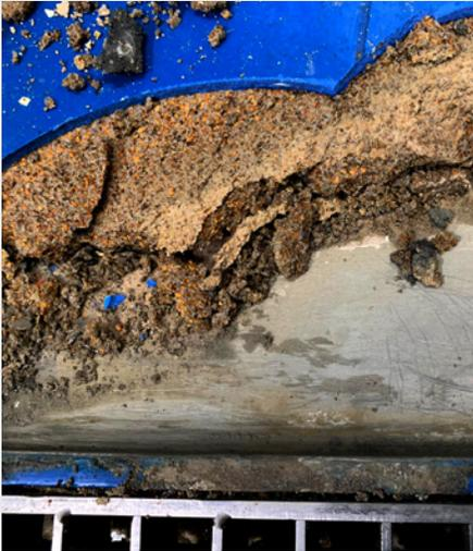
Water damaged and failed concrete underlayment adjacent to scupper.
