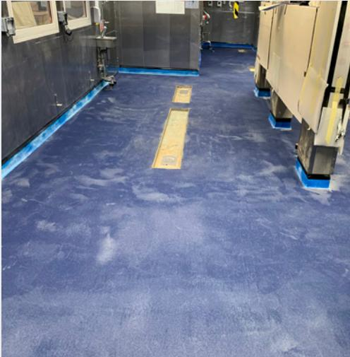
Installed SynDeck Flex IMO flexible, waterproof barrier epoxy with anti-slip quartz broadcast over waterproof resin underlayment.
