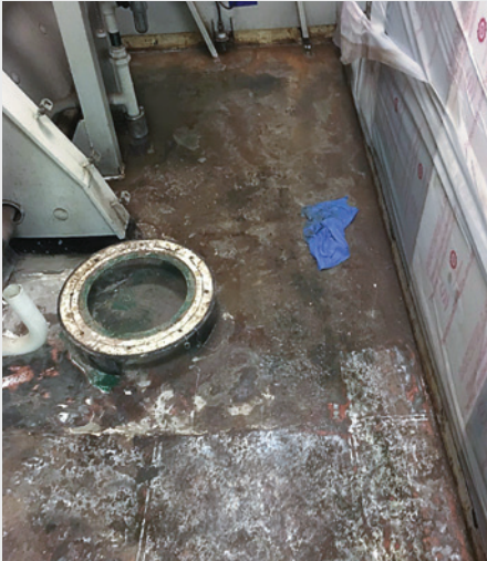
Extensive steel deck corrosion caused by water ingress through rubber tiles and concrete underlayment.
