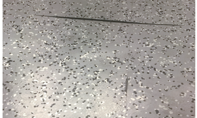
Delaminating rubber tiles in wet spaces due to water ingress at seams, creating significant safety and maintenance issues.
