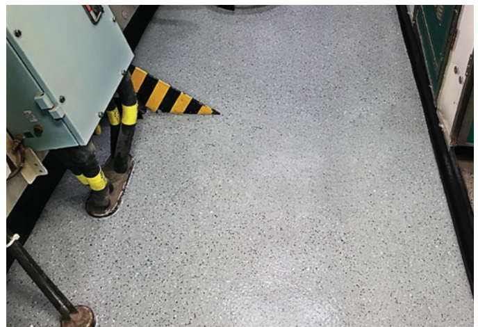
Installed wet space, decorative floor with SynDeck waterproof, seamless, full resin system.
