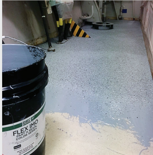
Installation of flexible, resin coating with flake broadcast over lightweight, resin underlayment in wet space.
