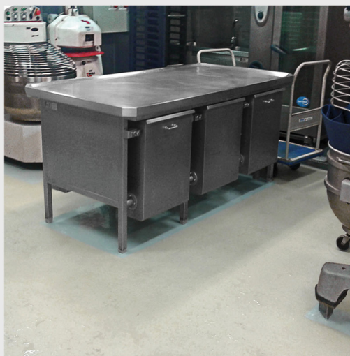
Completed anti-slip, full resin, galley decking system.
