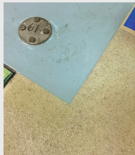
Detail of anti-slip finish for safety and smooth finish for easy cleaning.
