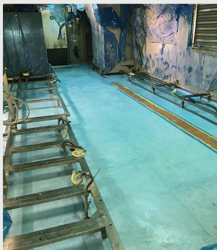
Installed SynDeck waterproof underlayment over galley deck with slopes to drains.
