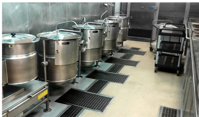
Installed galley floor with SynDeck waterproof, properly sloping, full resin system. Smooth finish under units in wash down areas.
